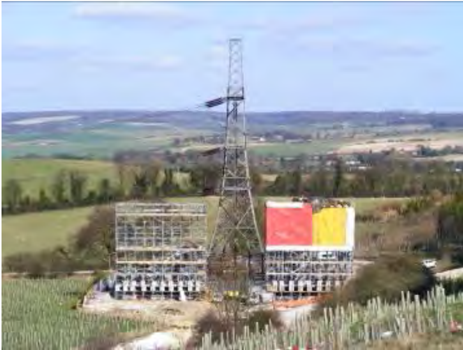
Figure 23 – Weatherproof enclosure for cable termination assembly
