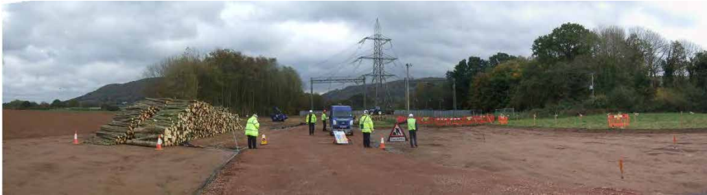
Figure 34 – Clearing woodland from the swathe (Ross-on-Wye 400kV)
