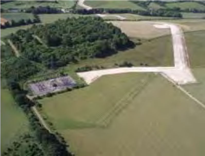
Figure 24 – Moulsoford Down 400kV SEC near Goring
