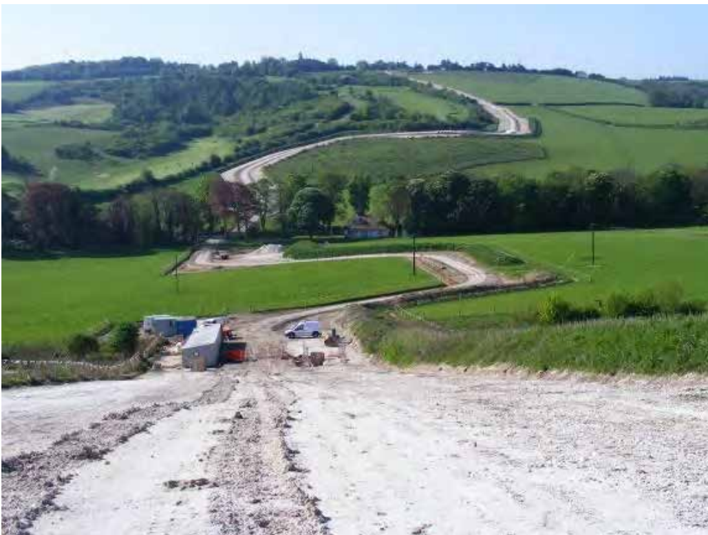
Figure 35 – 400kV cable swathe at the Goring Gap
