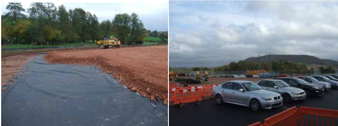
Figure 28 – Site storage/laydown area and site administration
