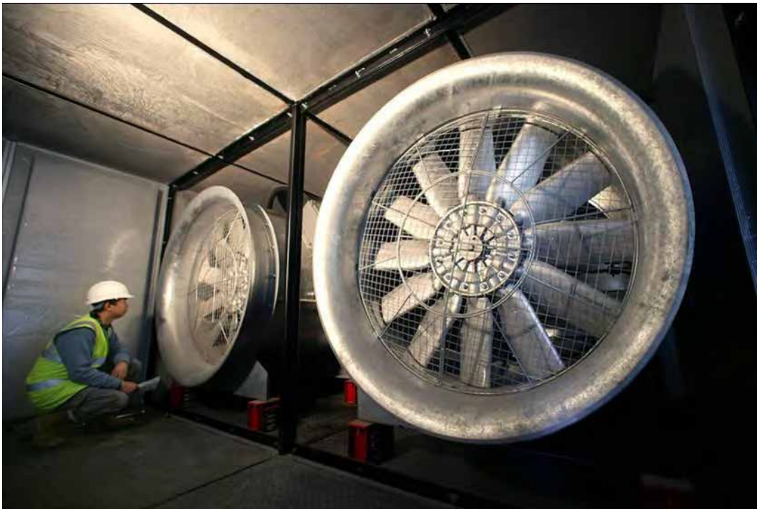
Figure 46 – Air cooling fans during installation
