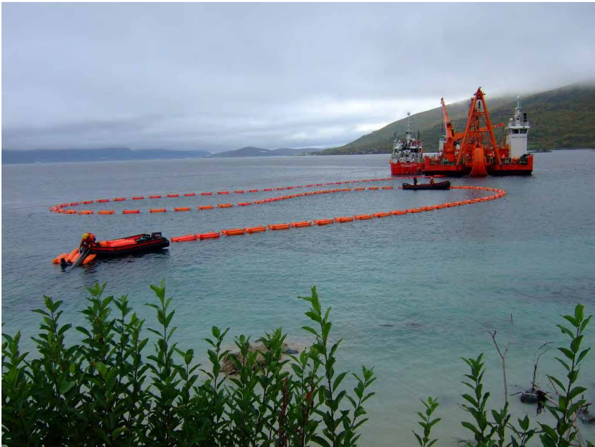
Figure 55 – Cable laying vessel shore landing installation
