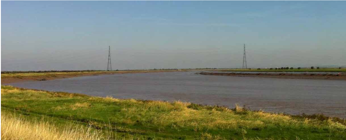
Figure 9 – Combwich Reach river crossing
