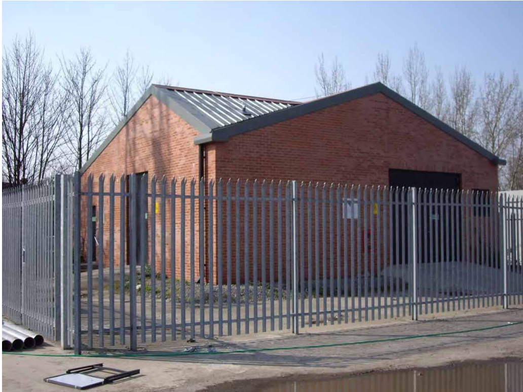
Figure 72 – Completed shaft head-house, within a secure compound
